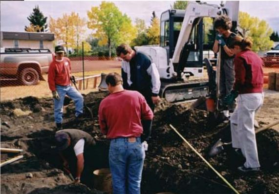
*The gravels turned to cobbles, impossible for the augur. We had to trench, and set forms to hold the concrete for each of the posts*
